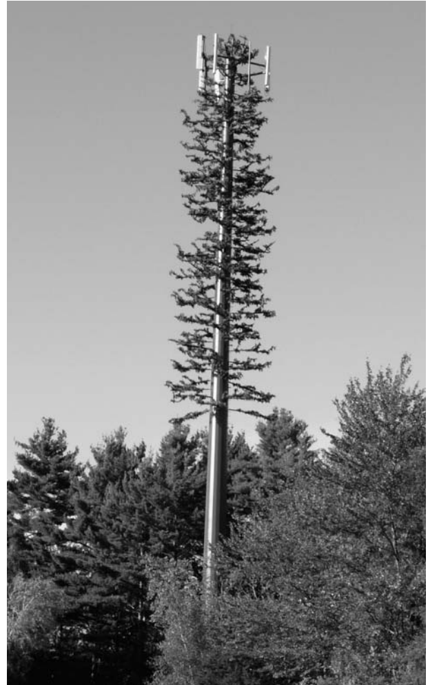
A cell phone tower disguised as an evergreen tree. Cell signals are sent through towers via radio signals.
