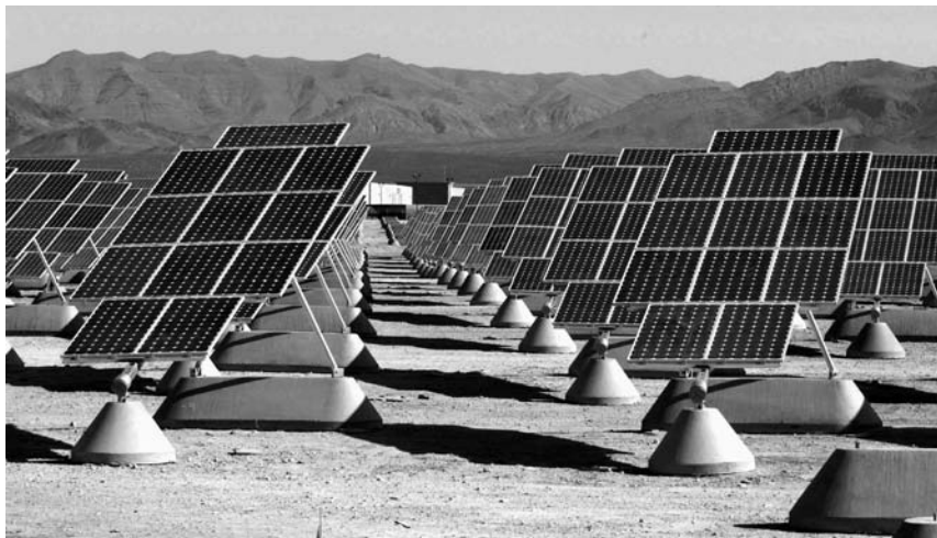
The solar field at Nellis Air Base in Nevada has more than 72,000 panels and supplies the base with more than 30 million kilowatt-hours of power.
